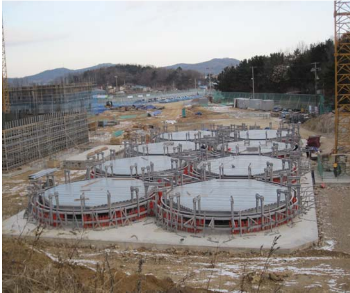
Ø12.0*40.5mH Grain SILO 8ea(Asan) – Seohee Construction 2010.
